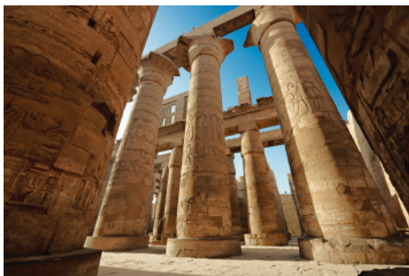
FIGURE 2.17. Central colonnade and clerestory windows in the Great Hypostyle Hall of Karnak. The great papyrus columns of the central aisle reach heights of 70 feet (21 meters). Alamy.
